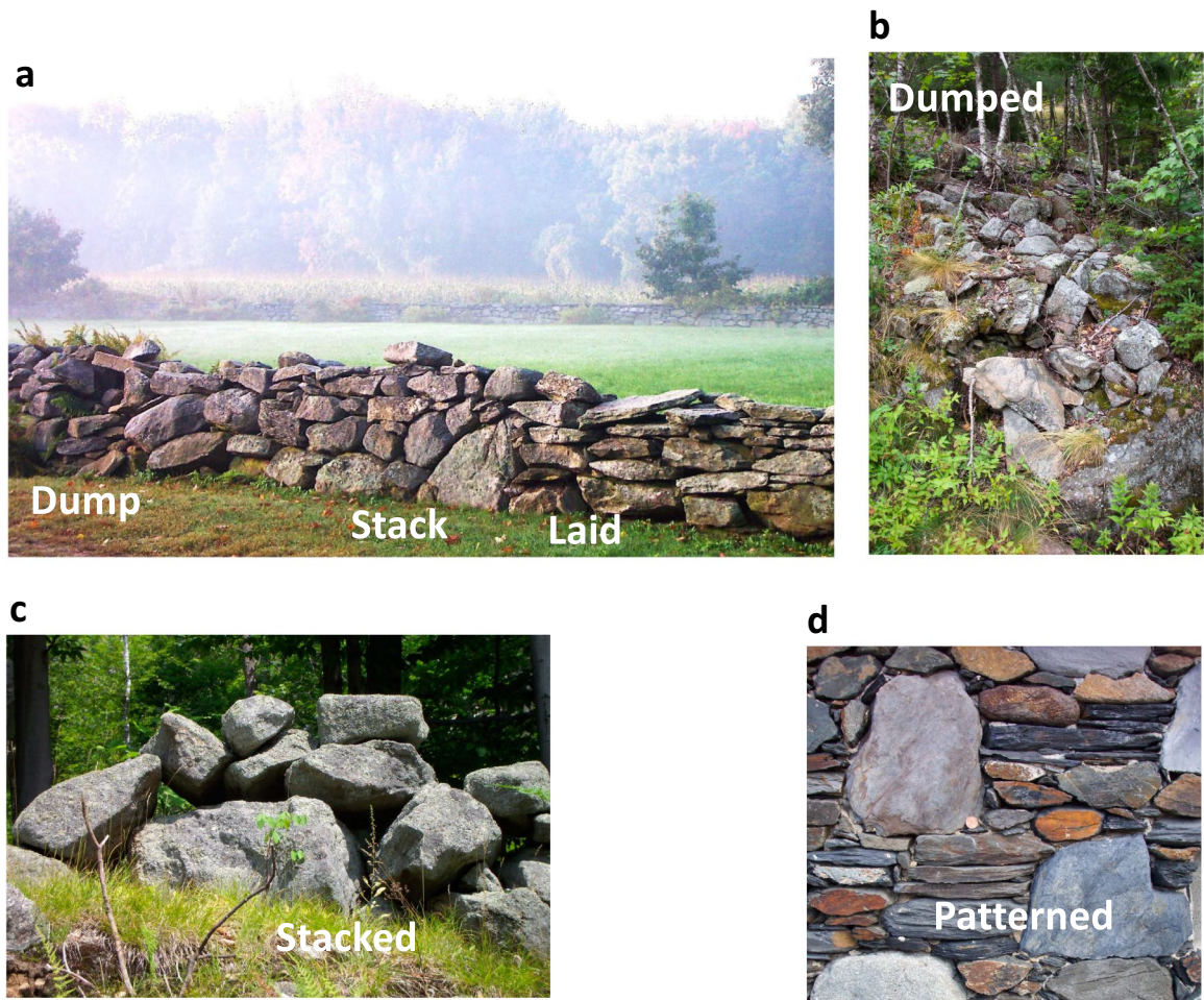
Fig. 9 Examples of degree of order in wall construction. (a) Single wall at Nathan Hale Homestead in Coventry, Connecticut, shows three segments defined by different degrees of order: dumped, stacked, and laid. (b) Wall in Weld, Maine, near the northern end of the common occurrence of New England walls is dumped, a characteristic of pioneering farm-
